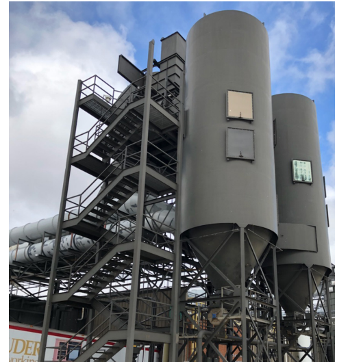
Dust collectors collect and filter our wood waste from manufacturing.
