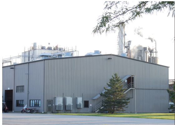
Sauder Co-Generation Plant
