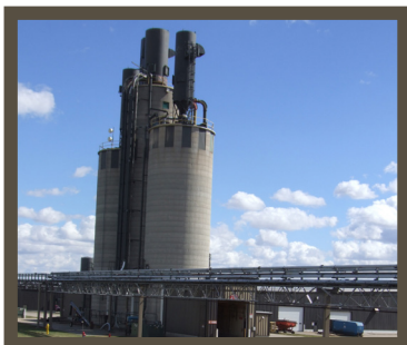
Sawdust is ground and stored in three main silos.
